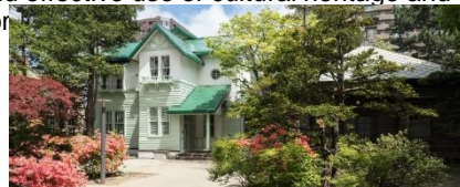
Former residence of Takeshiro Nagayama and former dormitory of Mitsubishi Mining Company, Sapporo City
