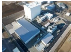
Biomass power generation station in Tomakomai City (put in service starting in February 2026)
