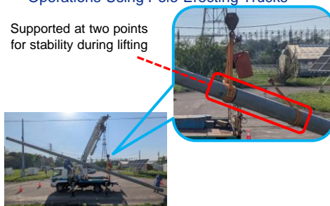
Improving the Efficiency of Hoisting Operations Using Pole-Erecting Trucks
