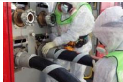
Training to replace the water supply in order to keep cooling the fuel
