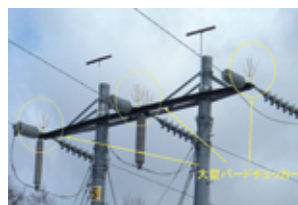
Bird checkers mounted on pylons
