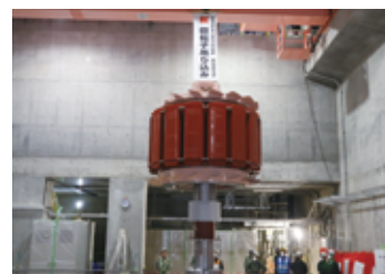
Retrofitting the generator at Shintoku Power Station
