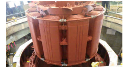
Retrofitting a generator at Sounkyo Power Station
