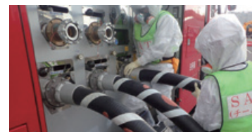
Training using alternative ways of supplying water to continually cool fuel
