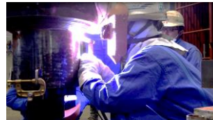
New welding method
