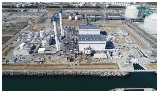
Unit No. 1 in operation (back) & Unit No. 2 in trial operation (front)
