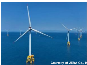
Offshore wind farm in Ishikariwan Shinko (put in service from January 2024)
