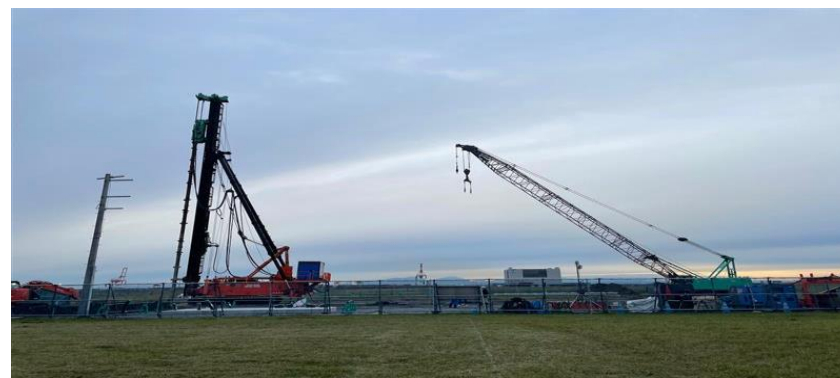
Status of construction (piling) as of October 11
