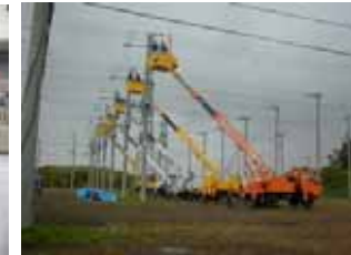
Exterior cabling training of the distribution department
