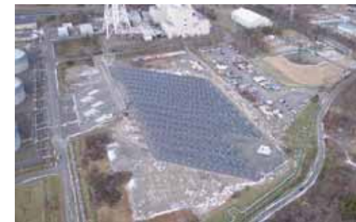
<Date Solar Power Plant> (under construction)
