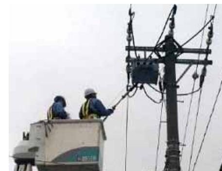
<Deterioration (flooding) test of the switch>
