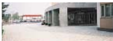
Execution example of permeable blocks
