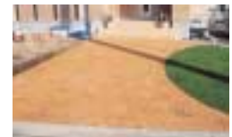
Example of Ash Brick being installed at a typical home
