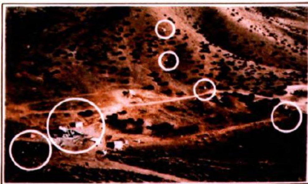
(b) Aerial View of Site after Rupture
